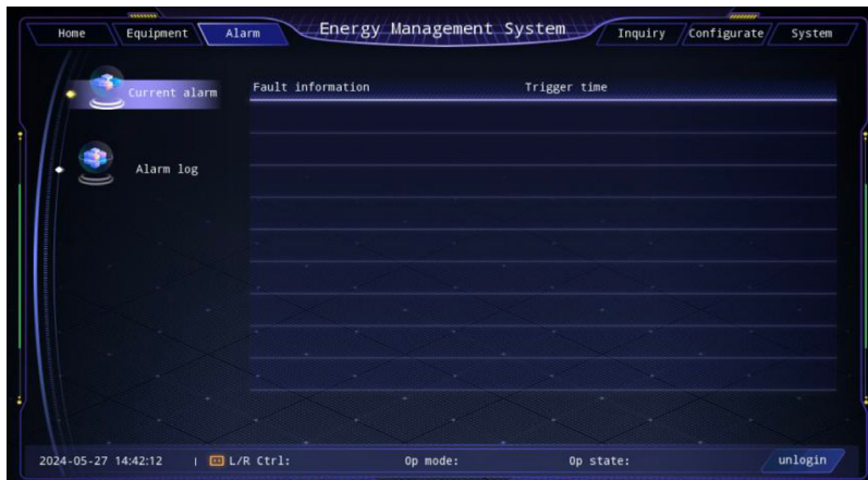
Figure 1.10 Real-time alarm information Interface
